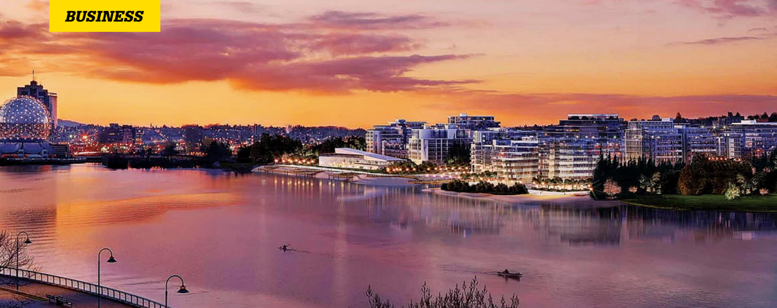
FEATURING 200 UNITS in South East False Creek, Millennium Water is being billed as Vancouver's last waterfront community
